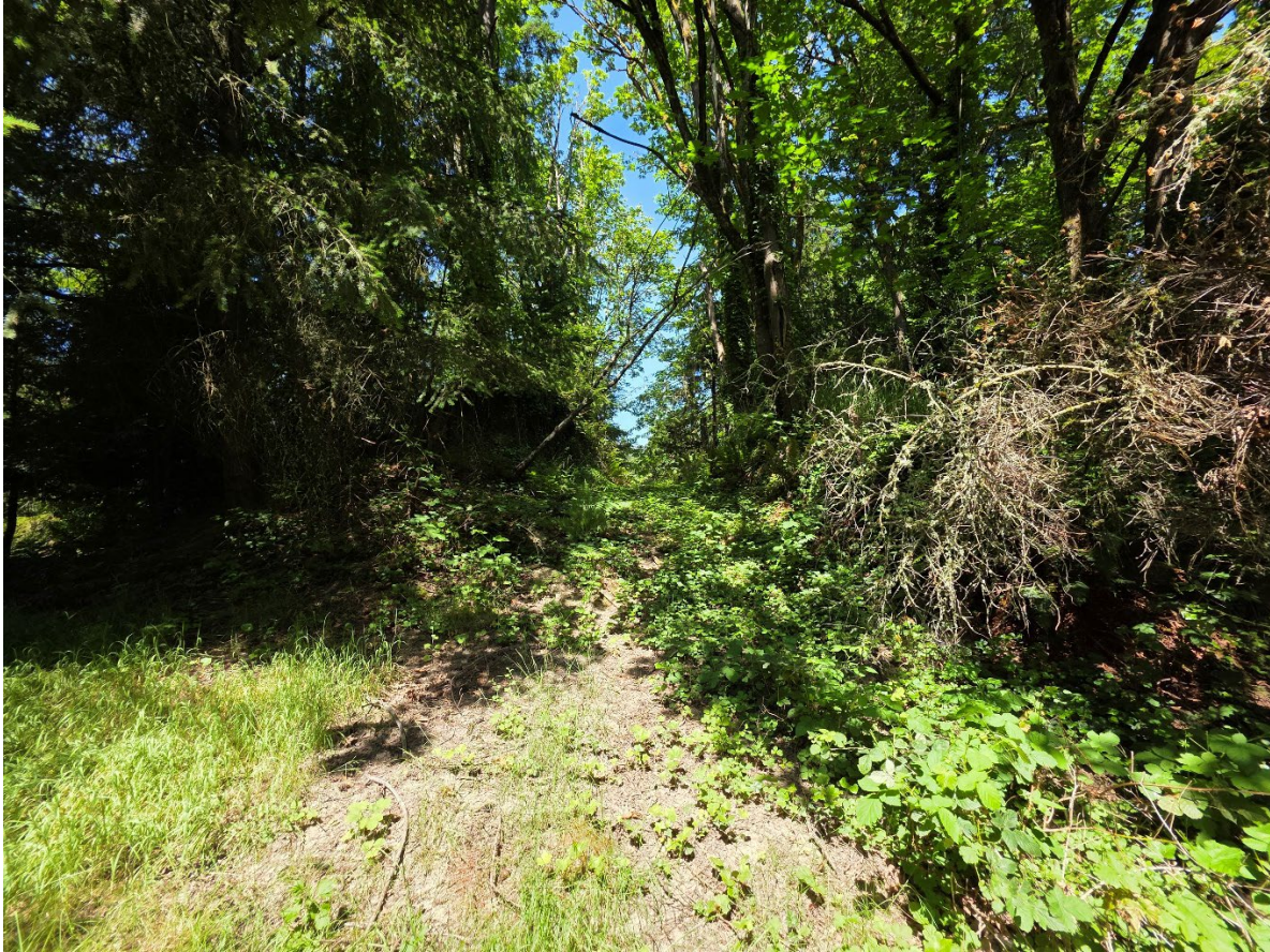
Plate 2 – “Road” cut, looking uphill to the west along the ridge crest. Note vertical slope in shadow on left. (6/18/2025)
