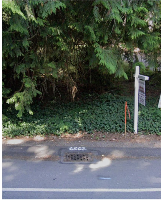
Photo 2 (looking west): type 1 catch basin. 12" concrete pipe flowing north.
